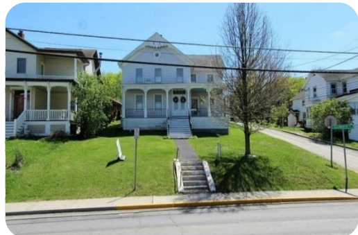
Single-family housing in the BOA on Main Street
