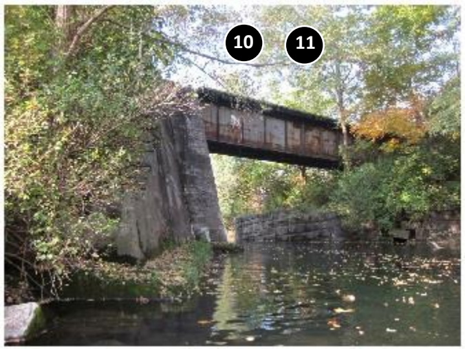
Strategic Sites 10 and 11, the train trestle and former rail bed, are located in Subarea 4
