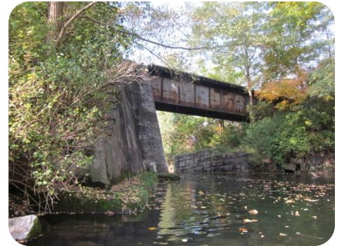
Philmont Reservoir Railroad Bridge
