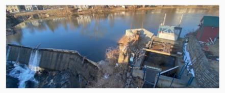
The environmental impacts and considerations of the facility were also discussed during the visit. Water flow over the dam and fish impacts were addressed, as was the importance of using trash racks with a 1" or less opening. Auto-cleaning trash racks were recommended to reduce maintenance requirements at the dam site. John also noted that there are extra permitting challenges if the waterway is a trout stream.
