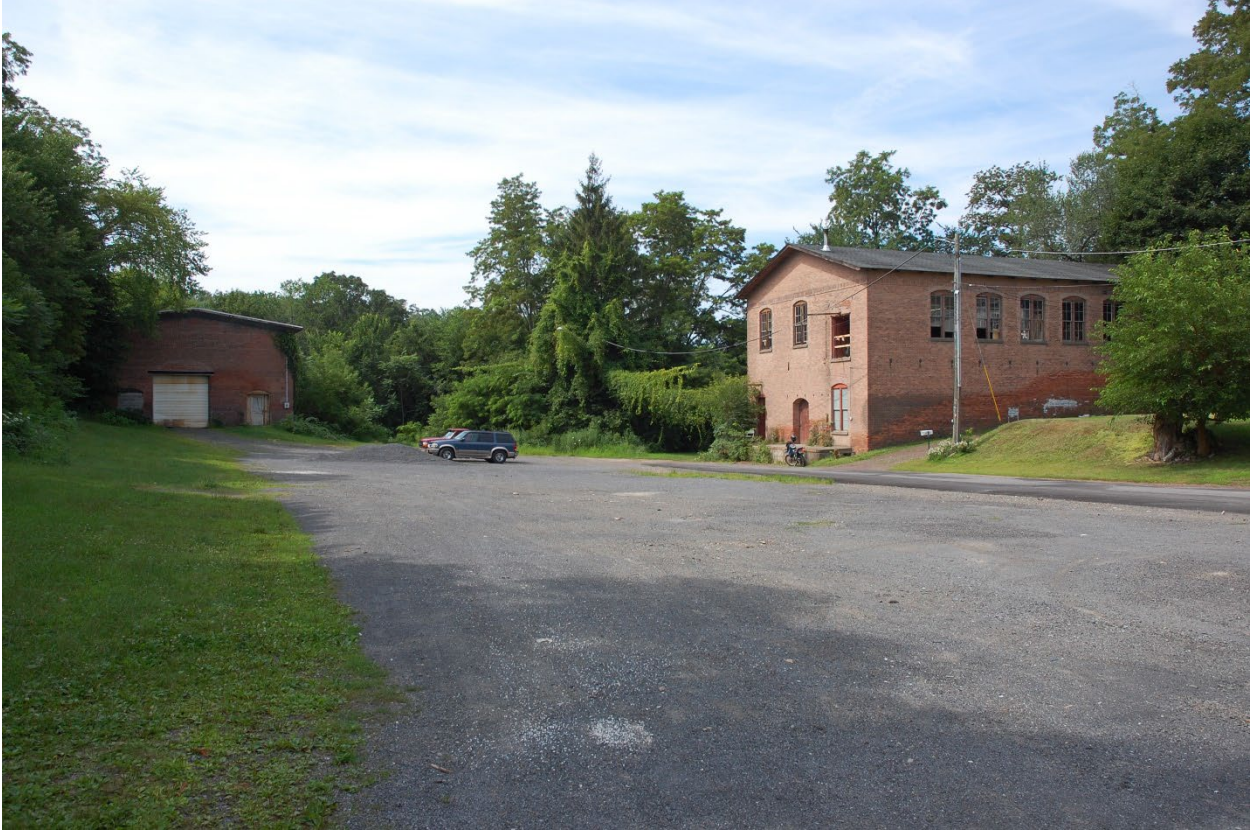
Canal St area
