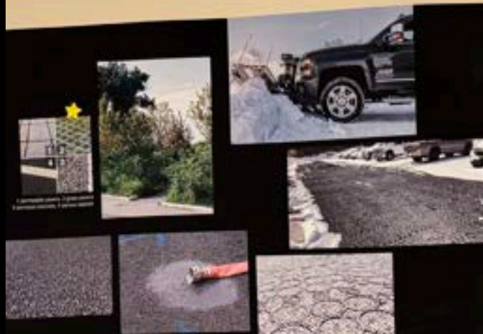
plowable, permeable parking surface within landscape chip seal, permeable asphalt, pervious concrete, blue grid pavers
